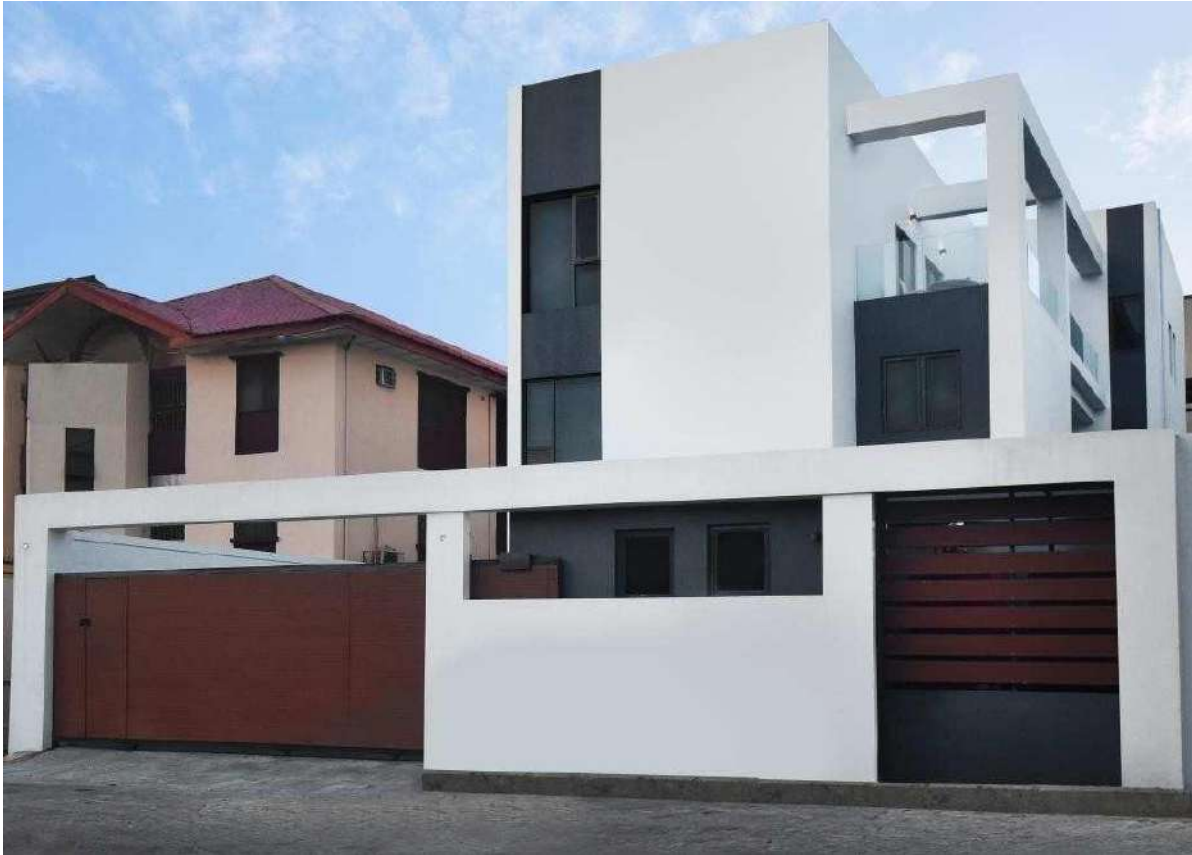
Image of Completed Residential Building for Mr & Mrs Ogunbiyi on Manuwa Close off Keffi Road (Project Cost =N300m)
